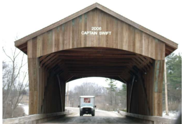
Captain Swift Covered Bridge (Kandace Tabern photo)
