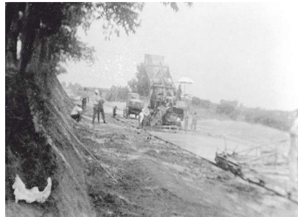
Construction of the Cannon Ball Trail (Public domain photo)
