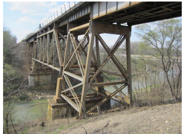
The old BNSF Bridge over Big Bureau Creek (Courtesy: Steve Conro)
