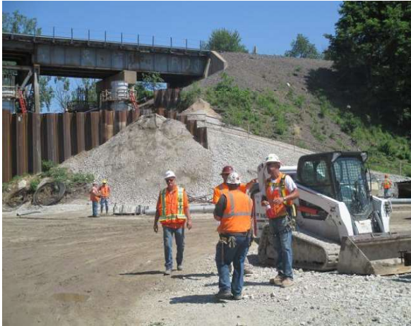
Construction crews working on a new bridge (Courtesy: LaSalle News Tribune)
