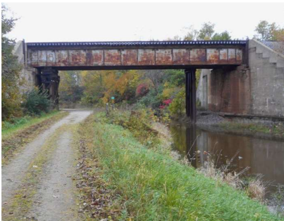
The BNSF bridge over the Hennepin Canal (Robert Tabern photo)
