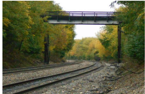
An old wood bridge, east of Buda on the BNSF (Robert Tabern photo)
