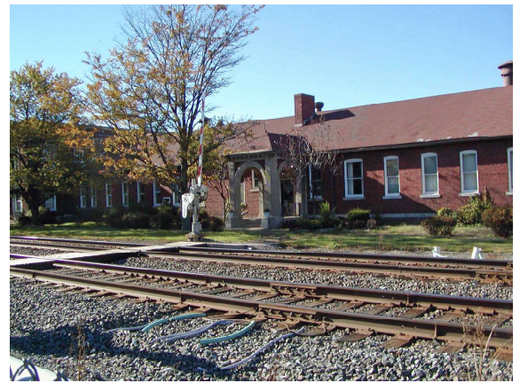
Former Kewanee Boiler Co. administration building.
