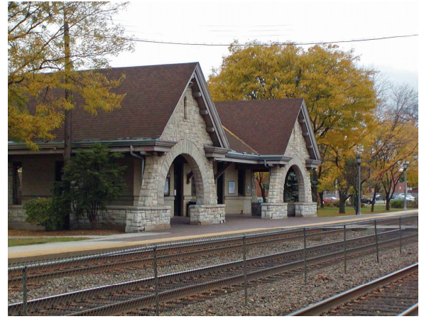
La Grange's Stone Ave. Depot.
