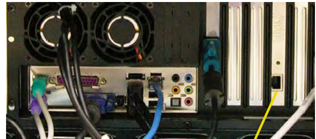
External Ethernet Connection
