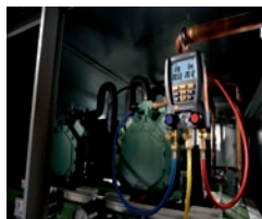
Conduct leak test
