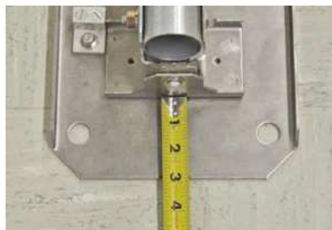
Figure 28: Tape Measure in Slot for South Anchor
