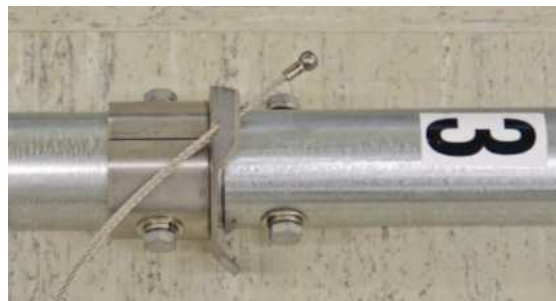
Figure 19: Mast Section 3 and Guy Ring/Collar Assembly
