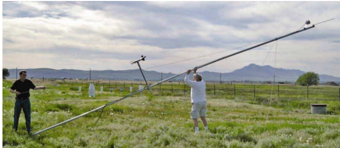
Figure 34: Raising the Mast.
