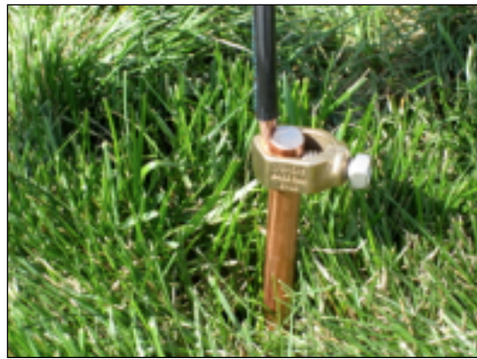
Figure 39: Grounding Rod Driven into Ground with Grounding Cable Secured
