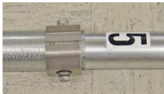
Figure 22: Mast Section 5 Installed in Mast Section 4
