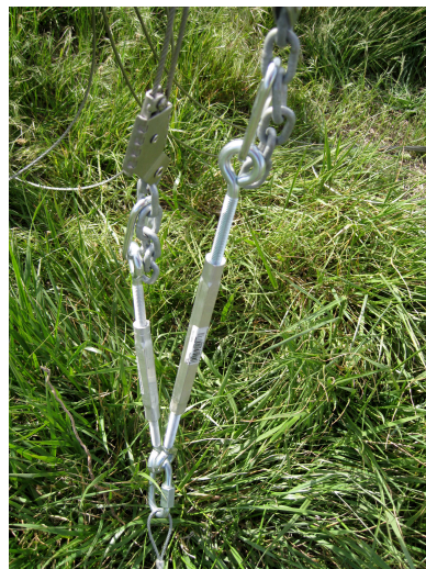
Figure 36: Adjusting Turnbuckles.
