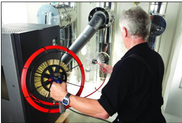
Fig. 20: Cleaning a stainless steel chimney
