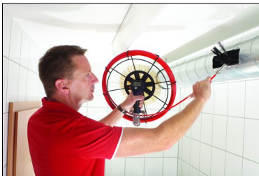
Fig. 21: Cleaning a ventilation duct
