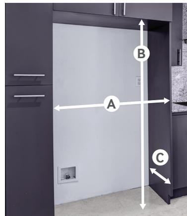
**A)** Measure height including flooring. Be sure to allow for hinge clearance height if needed.
